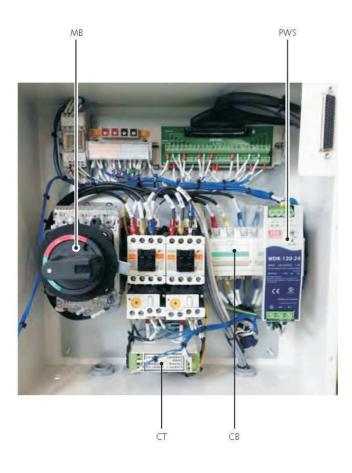
MB On/ off switch/ Main circuit breaker
